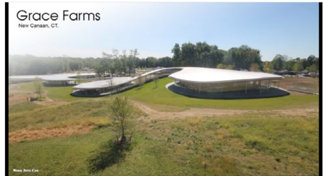
Watch construction of The River at Grace Farms in New Canaan with Work Zone Cam's time-lapse movie. The construction webcam captured progress for this beautiful project from September 2013 to October 2015, which can be seen in just 80 seconds. Video Credit: WorkZoneCam
